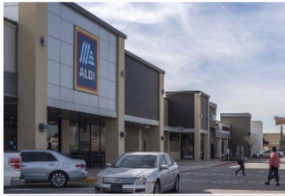
Tanglewilde Center Houston, TX
